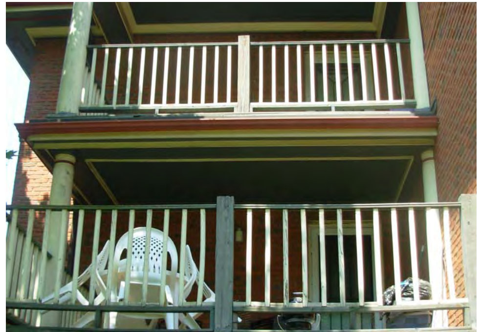
6. Wood-framed balconies exhibit deterioration
