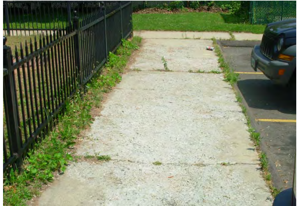
2. Cracking and spalling concrete walks
