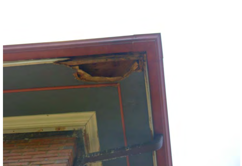
12. Soffit deterioration observed
