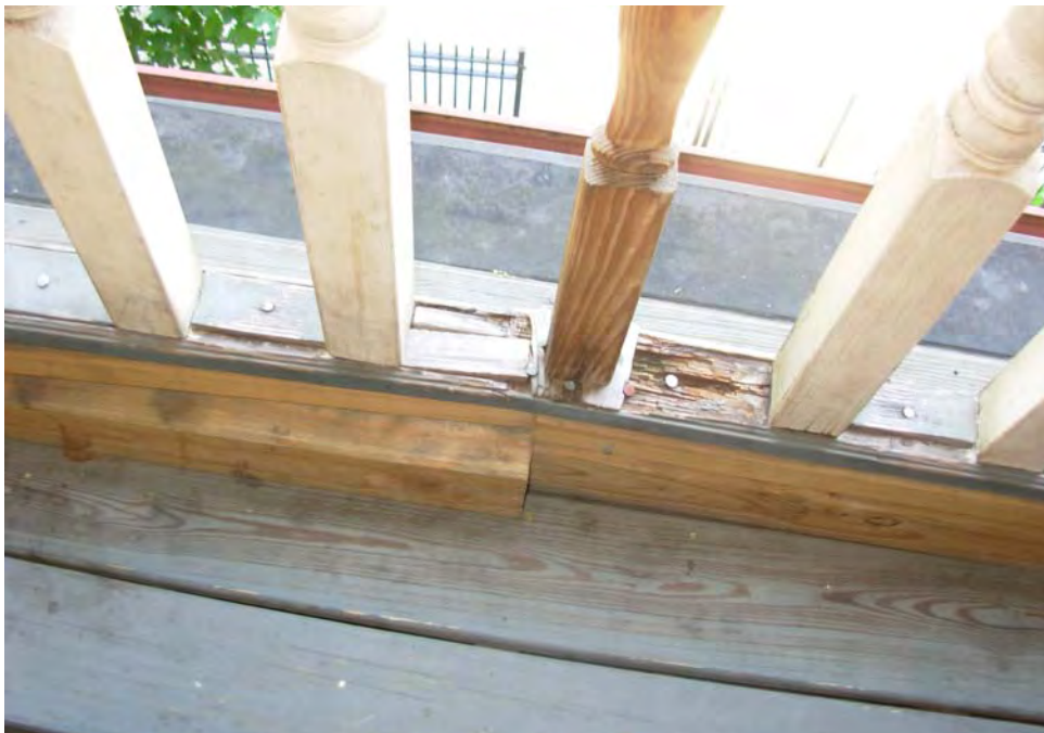
7. Wood railing deterioration at balconies
