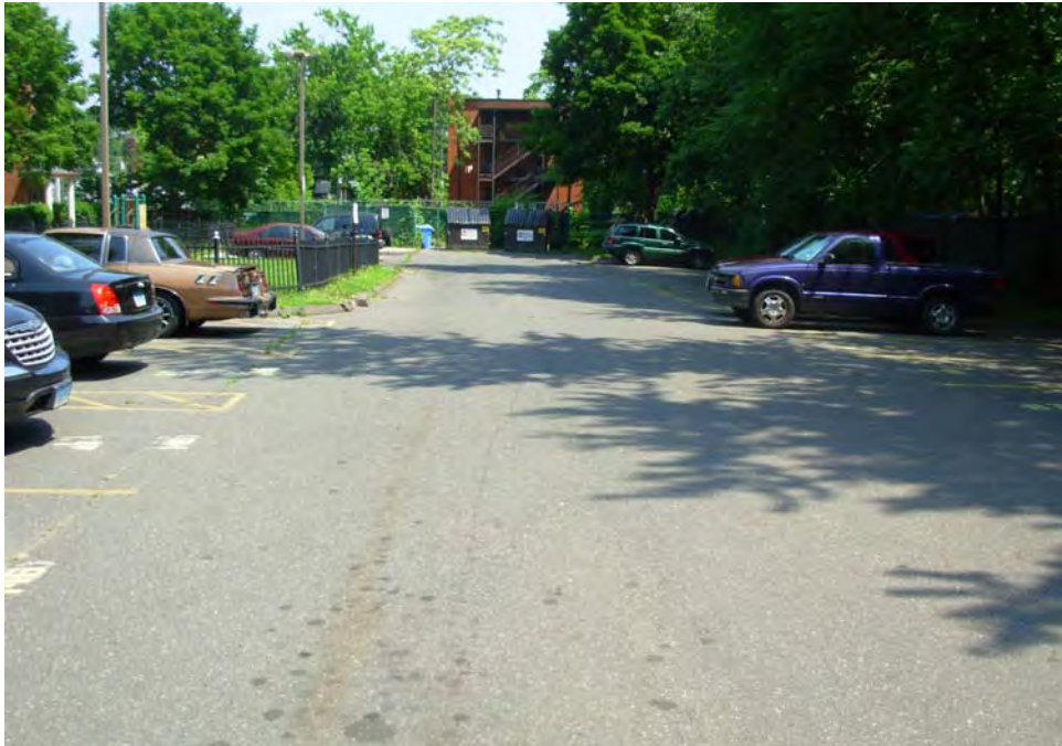
1. Parking area surfaces, cracking and settlement
