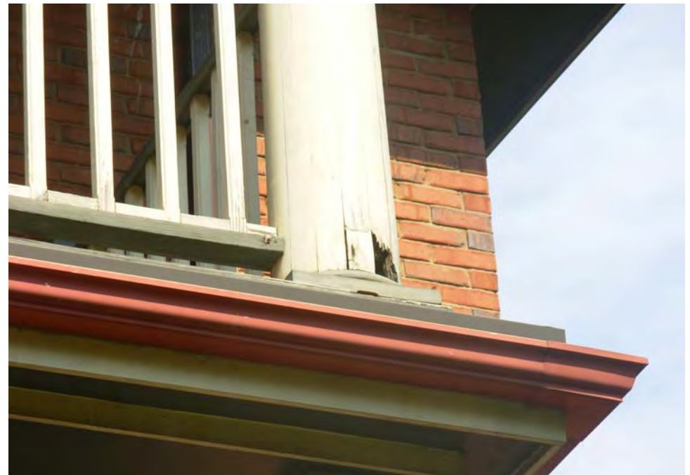
8. Support post deterioration at balconies
