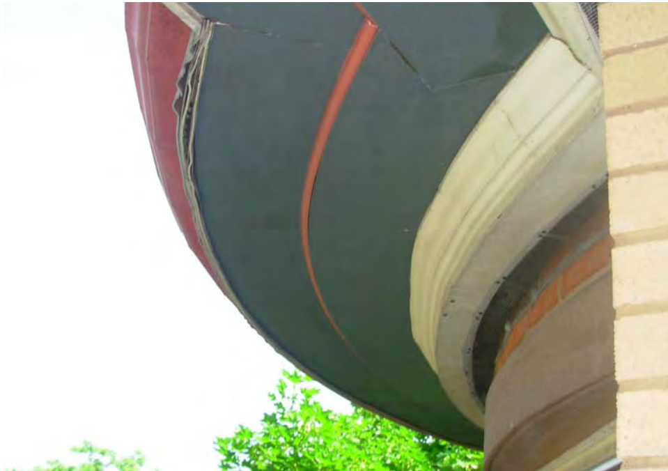
11. Fascia boards delaminating at front cornice sections
