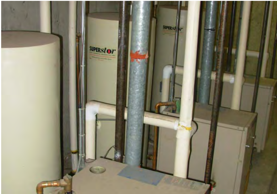
15. Heating and DHW generation equipment in basements
