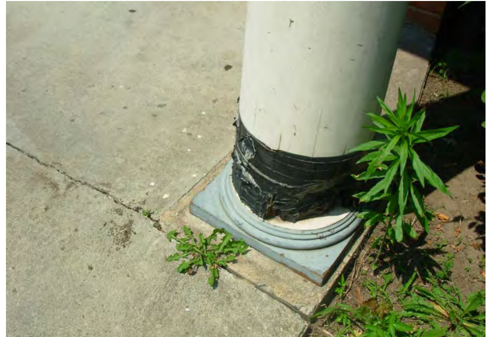
10. Wood support post deterioration, to repair and paint
