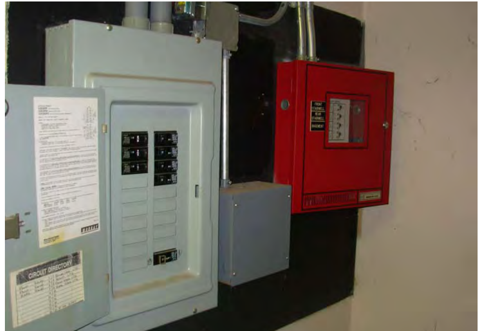
16. Main electrical panels and fire monitoring panels
