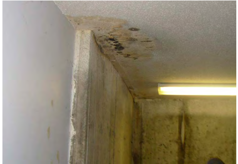
14. Water leak damage at basement level areas, some mold growth
