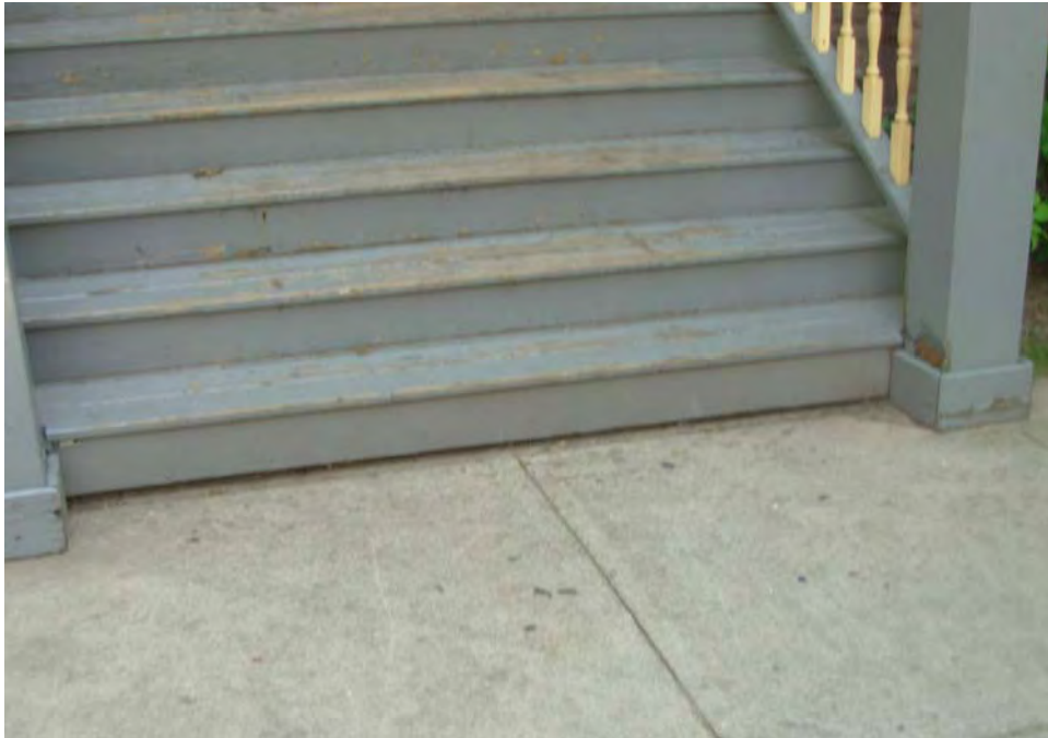
9. Wood front porches at each building, deterioration prevalent
